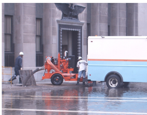
BGE Crew Hard at Work
