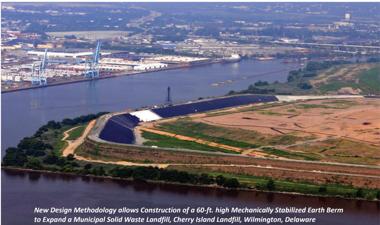
*New Design Methodology allows Construction of a 60-ft. high Mechanically Stabilized Earth Berm to Expand a Municipal Solid Waste Landfill, Cherry Island Landfill, Wilmington, Delaware*
